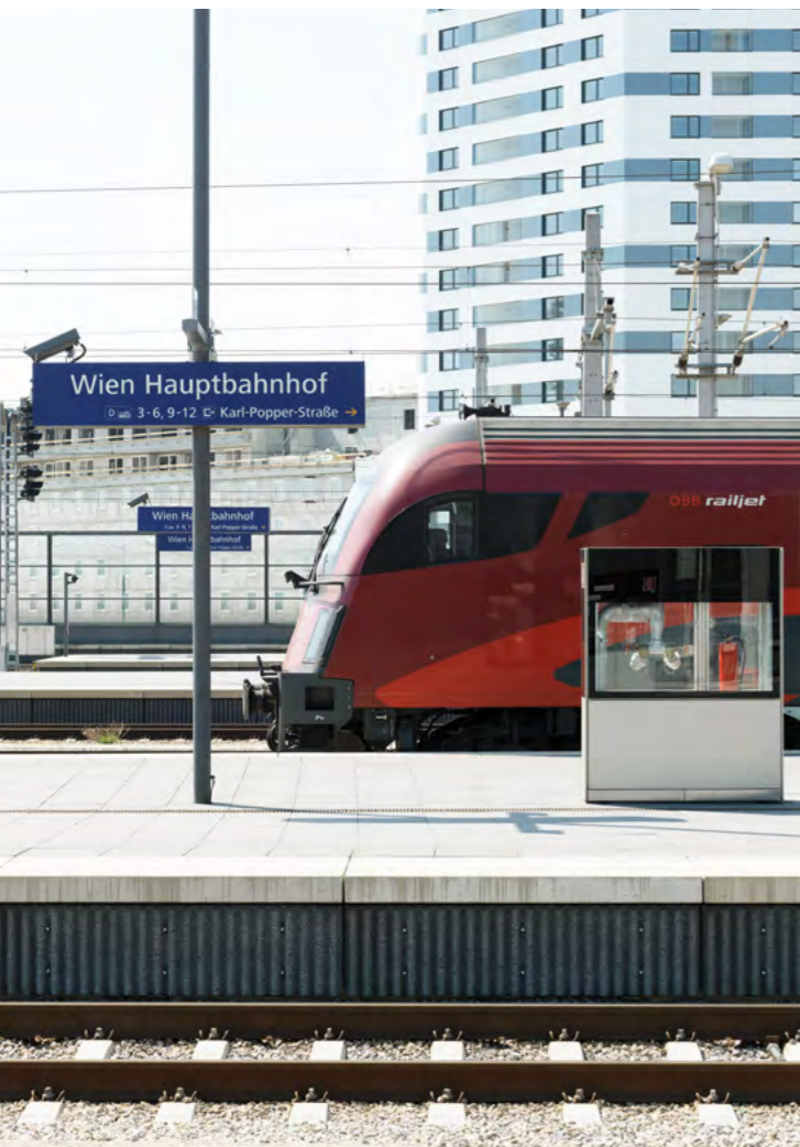
Highly absorbent platform edge, Vienna Central Station, AT
