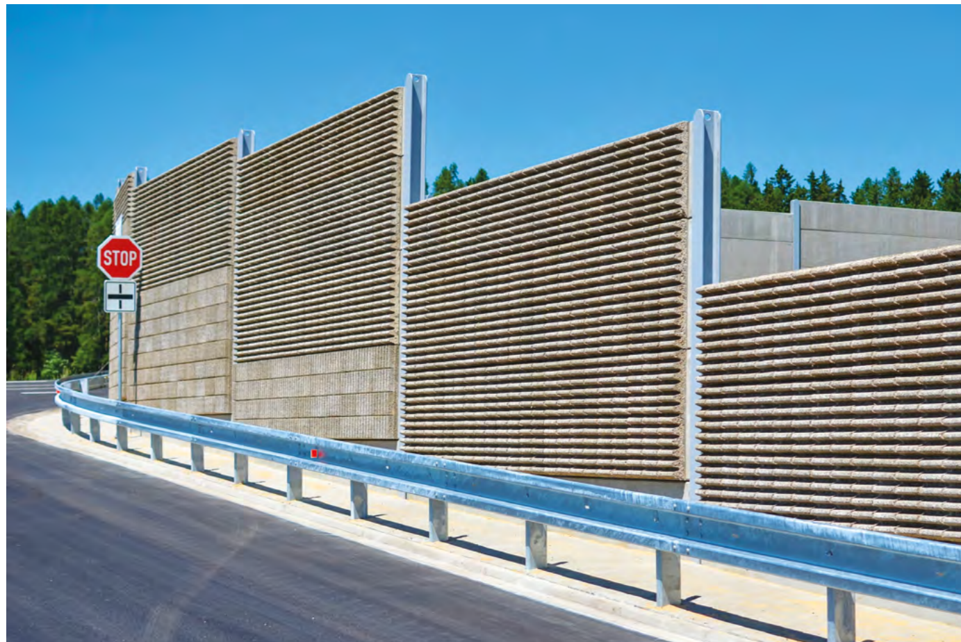
Road Noise-Protection System with Wave absorbers
