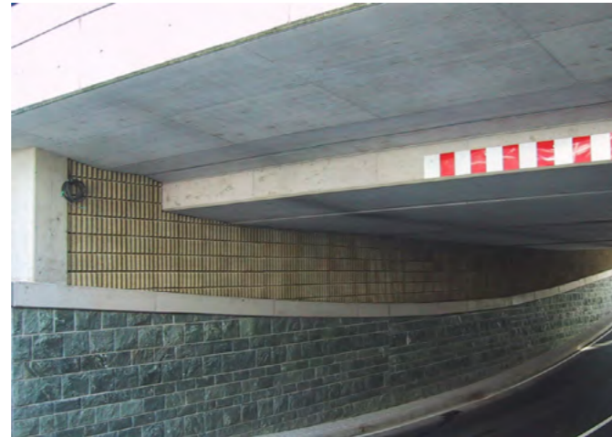
Cladding of a curved wall with Leube Faseton® Elements
