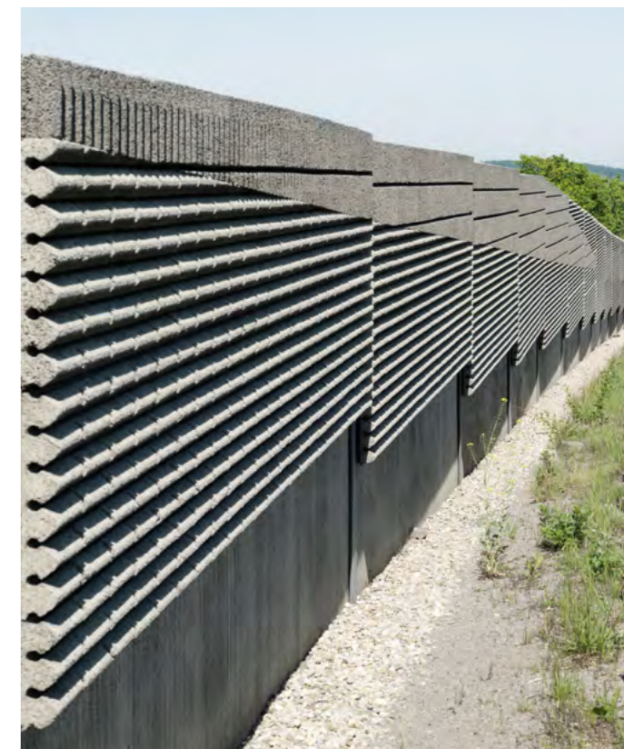
Straight Wall with Hollow Wave A1 West Motorway, Steinhäusl, AT
