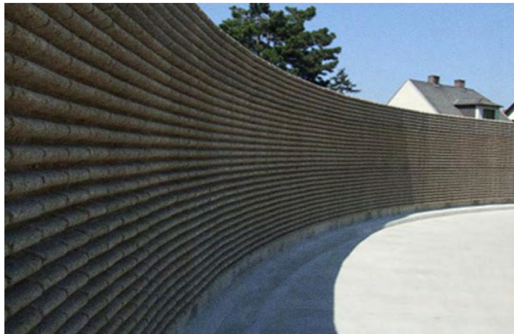
Cladding of a curved wall with Leube Faseton® Elements
