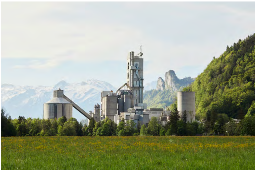
The cement plant on the Königsseeache river in Gartenau is the backbone of the Leube Group.
