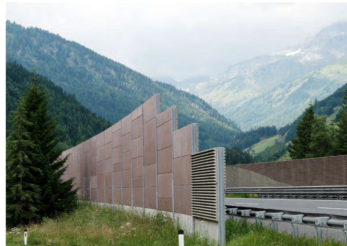
Backside design on the motorway
