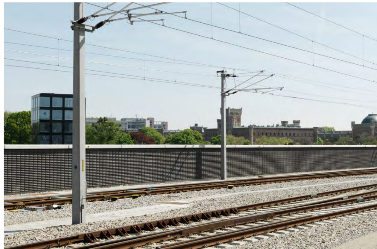
Wave for railway bridge, Vienna Central Station, AT
