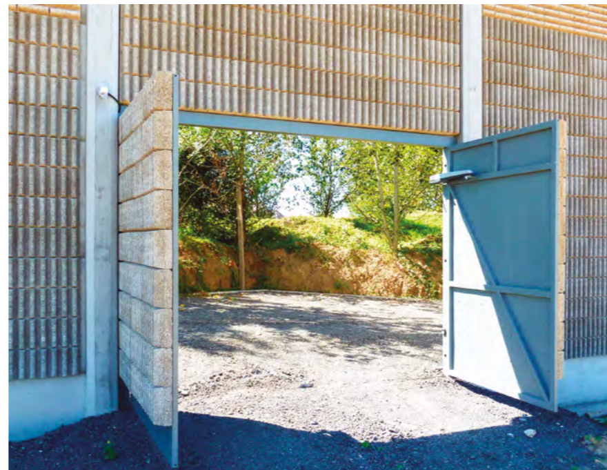
Cladding of door overhangs
