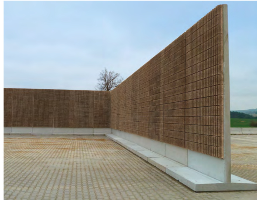
Cladding of concrete components
