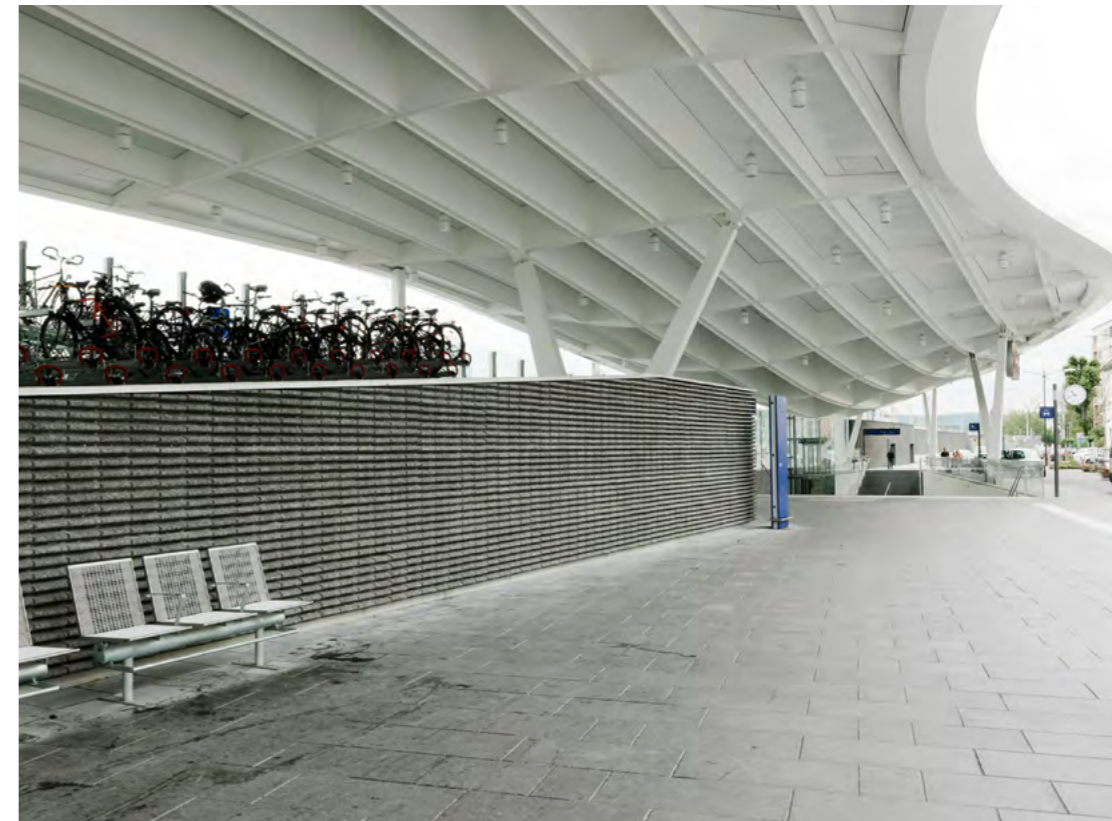
Wall cladding with Wave, Salzburg Main Station, AT
