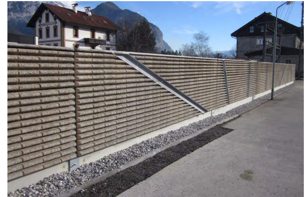
Steel U-shapes as a design component, Zirl Railway Station, AT
