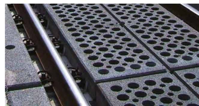
The Rieton track absorber is laid between the tracks.
