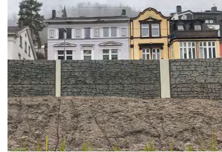
Backside cladding at Altona Railway Station, DE
