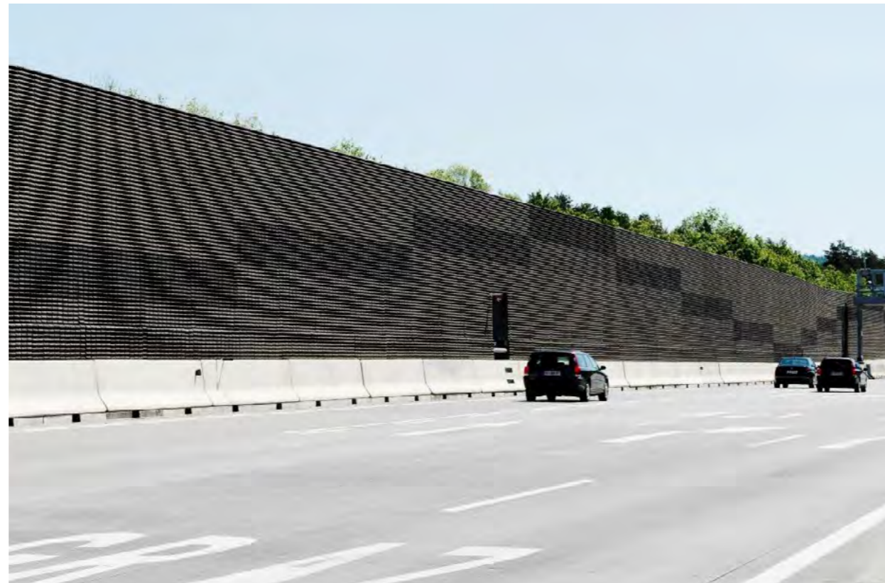
Straight Wall with Hollow Wave A1 West Motorway, Steinhäusl, AT
