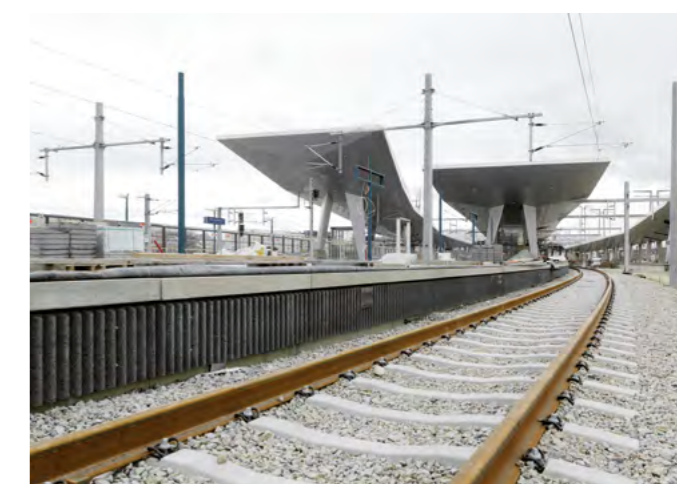
Highly absorbent platform edge, Vienna Central Station, AT
