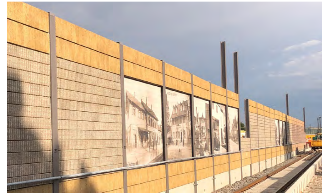
Backside design of Haltingen Railway Station, DE
